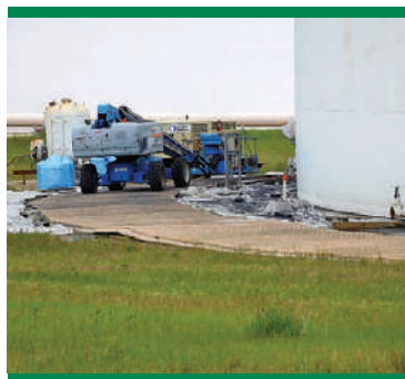
Maintenance Project in Louisiana
