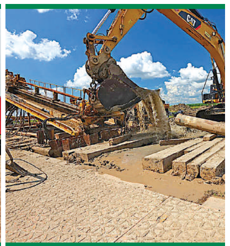
Directional Drilling Under Mississippi River
