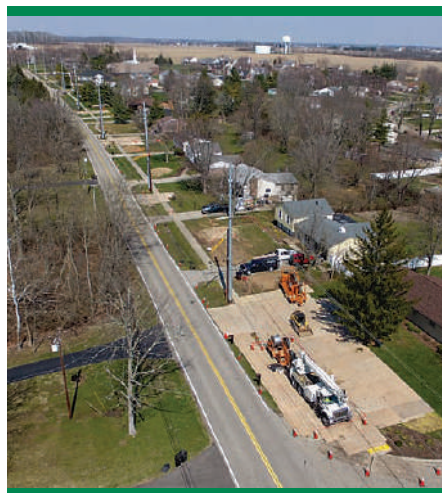
Access Road to Transmission Line Project
