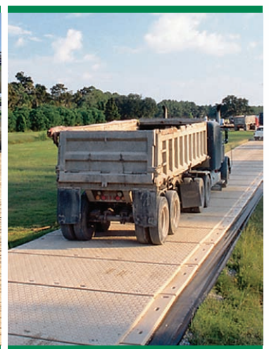
Temporary Road to Rig Platform
