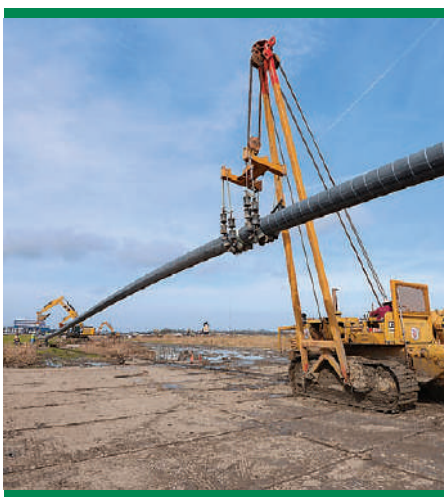
Pipeline Construction Project
