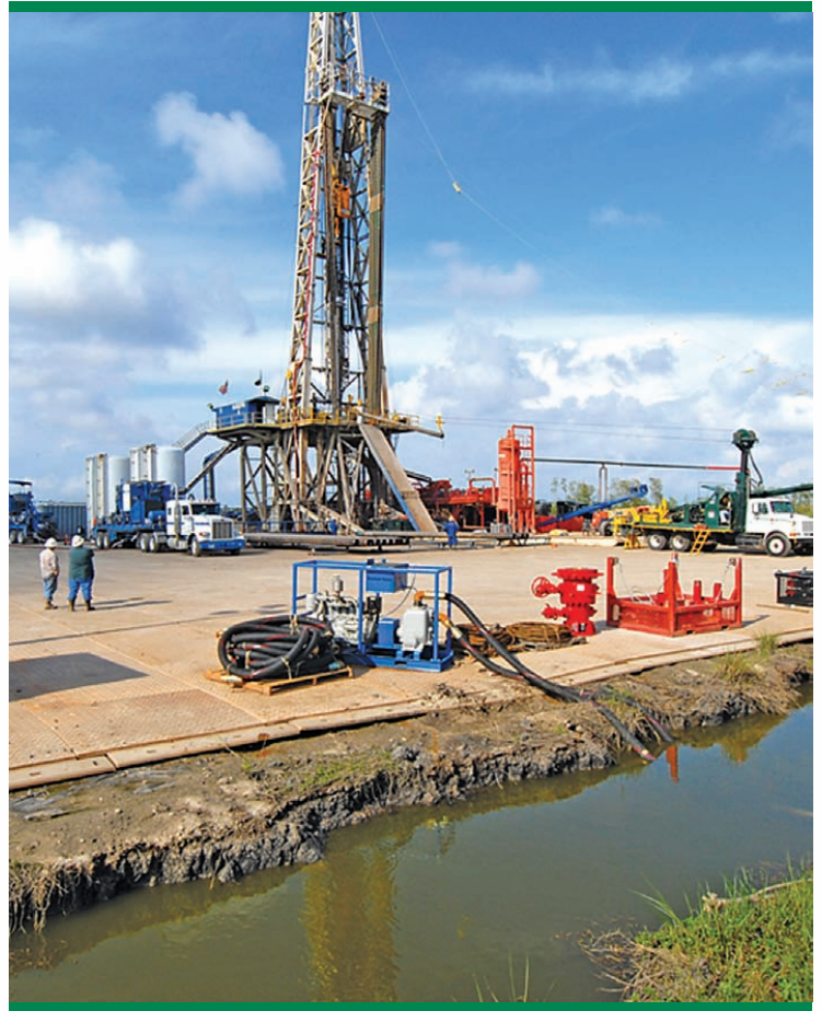
Solid Surface for Heavy Equipment at Drilling Site
