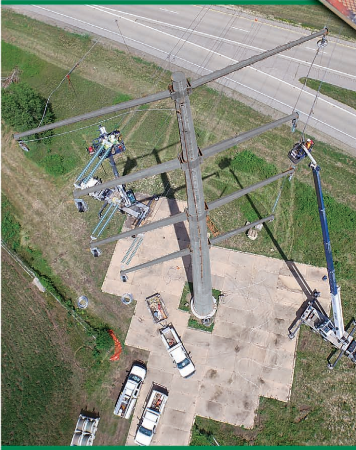
Stable Platform for Utility Projects
