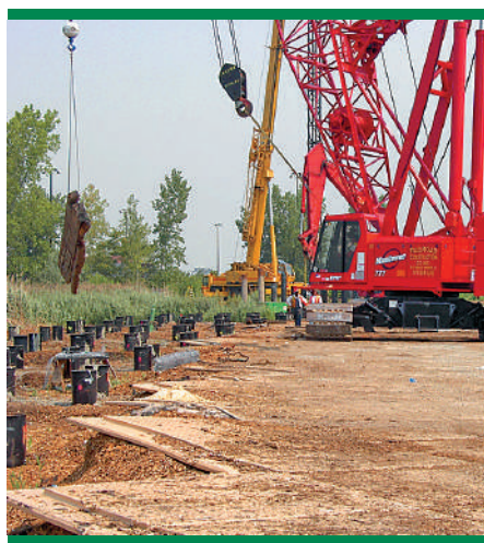
Pile Driving Project
