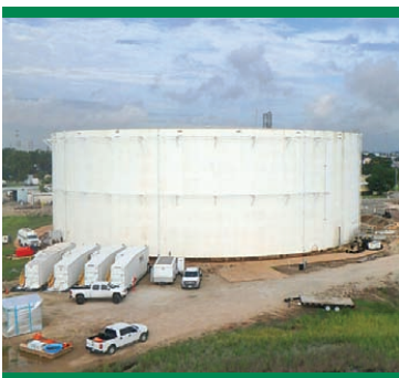
Tank Farm Project
