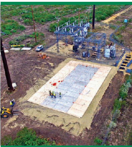
EPZ Grounding System on a Transmission Line Project
